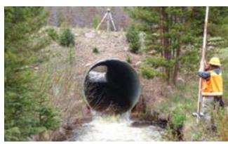
their native streams. While cost considerations are usually the dominant factor in determining what types of culverts should be installed, accommodations (flow, water level) for fish migration can be aligned with plans to prevent structural damage to the infrastructure. Intense precipitation events, nota-
