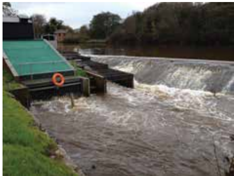
Larinier Fish Pass entrance with hydropower active.
