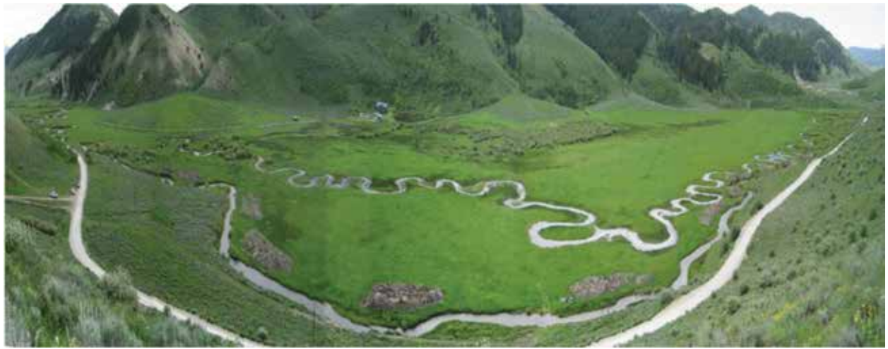
Figure 5. Photo of Crow Creek, Idaho, project immediately after we began to divert streamflow from the straightened channel (adjacent to road) into the reconstructed channel (top).
