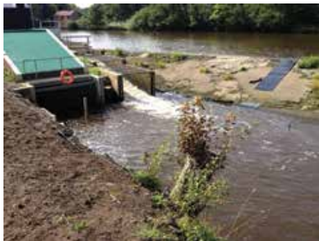
Larinier Fish Pass entrance with hydropower inactive.
