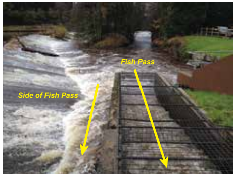
Fish pass & side-of-fish-pass ascent routes, downstream.
