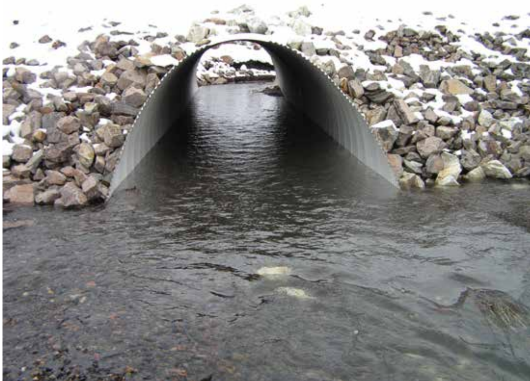
Figure 2. Culverts in Beaver Creek that prevented fish passage (top) were replaced with a fish-friendly structure in 2005 (bottom). Photos courtesy of Elko District BLM.
