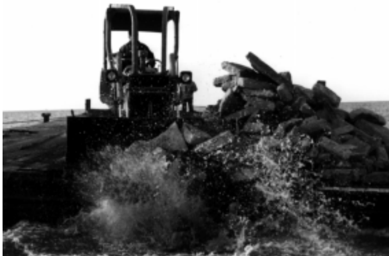
FIGURE 4.—Flat-topped barge and front-end loader used at the Lorain and Lakewood artificial reef sites to better control placement of reef materials. (Photo courtesy of D. O. Kelch, Ohio Sea Grant.)
