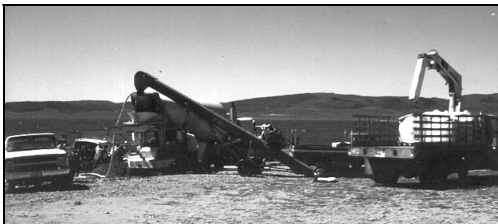
Figure 2. Slurry mixing system using cement truck.
